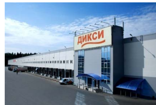
DIXY Distribution Center
